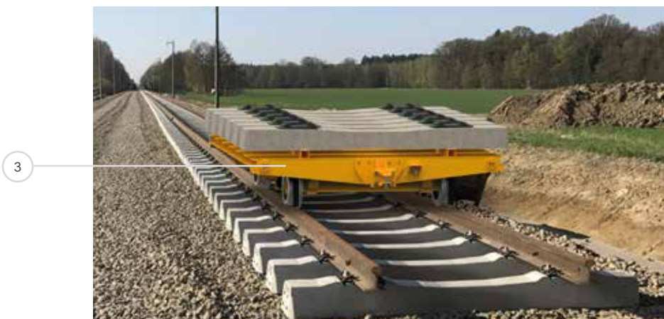
1. Sleeper Layer with fast clip module
